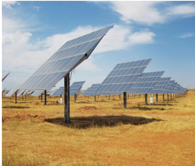
PV power plant planning works at MediaBroadcast Shortwave Station in Wertachtal, Germany
